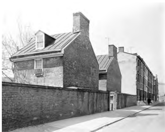
Workman Place. Note 'GM' (for George Mifflin) and construction date '1748' on the walls.
